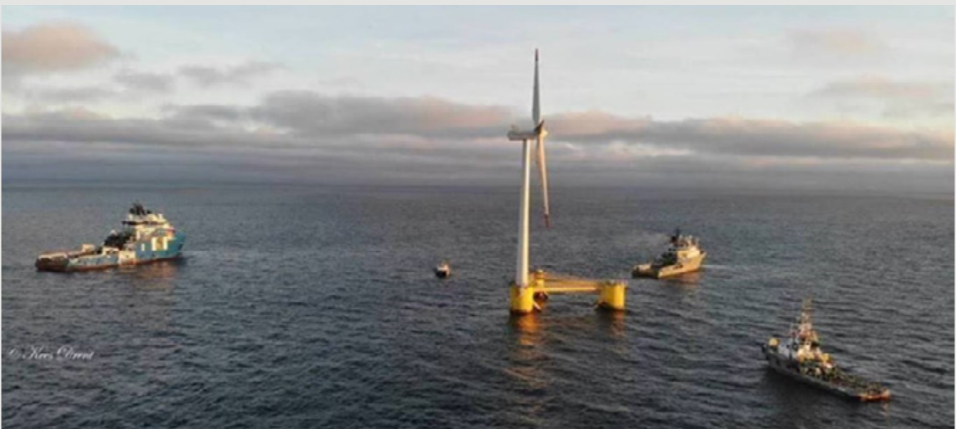
Fig 1: the Kincardine floating wind project: WGT tow-out
